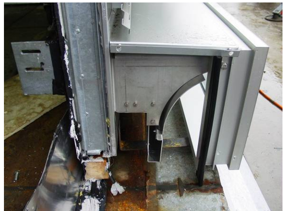
Fig. 24 Substructure with metal sheets at base point
