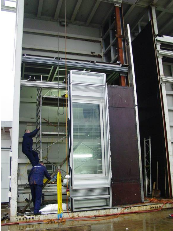
Fig. 21 Disassembly of test specimen
