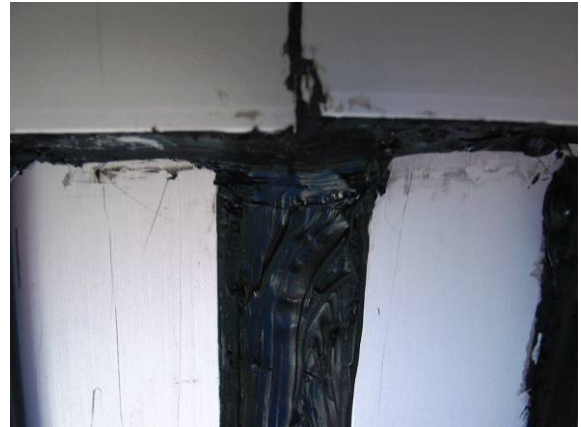
Fig. 18 Joints sealed internally with elastic sealant
