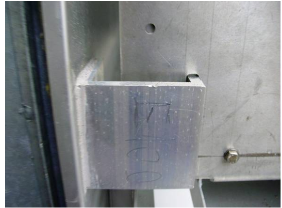
Fig. 26 Hook-on, fixing brackets of secondary facade
