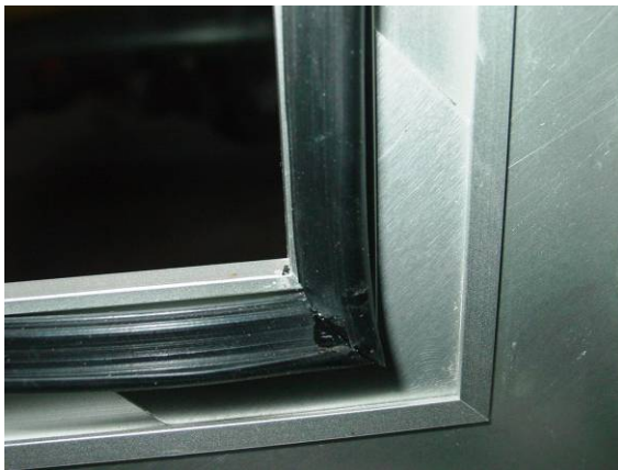
Fig. 7 Corner design of casement rebate seal
