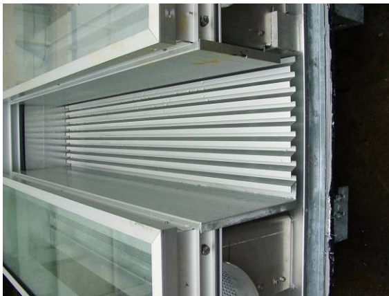
Fig. 27 Lamella grating between double skin facade
