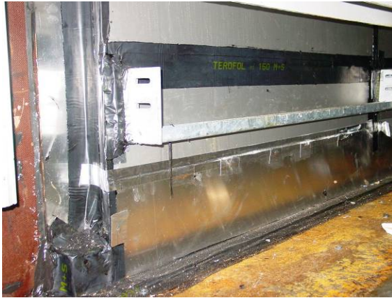
Fig. 17 Coupling joints internally masked with sealing membrane Terofol (M+S) vapour tight
