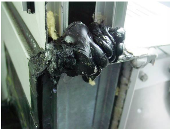
Fig. 23 Sealing of primary facade at coupling
