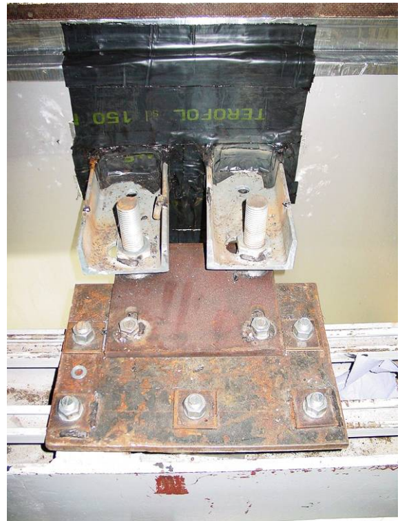
Fig. 20 Fixing brackets internally masked with sealing membrane Terofol (M+S) vapour tight
