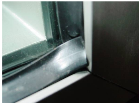
Fig. 8 Corner design of external glazing gasket
