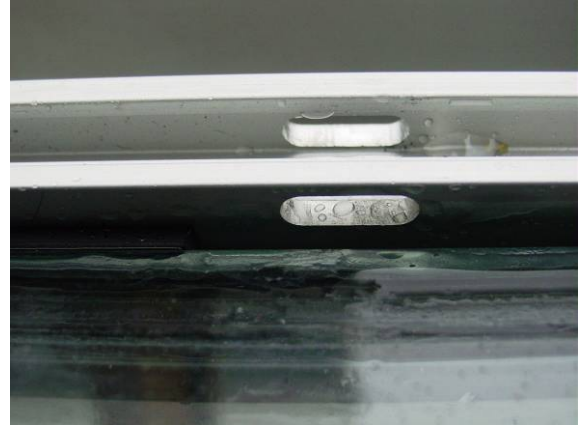
Fig. 12 Rebate drainage
