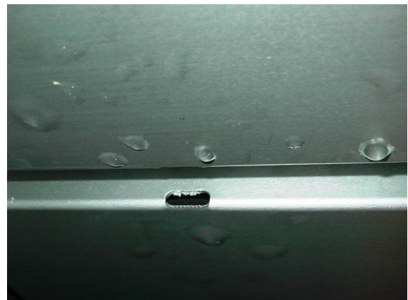
Fig. 14 Drainage slot in facade cavity
