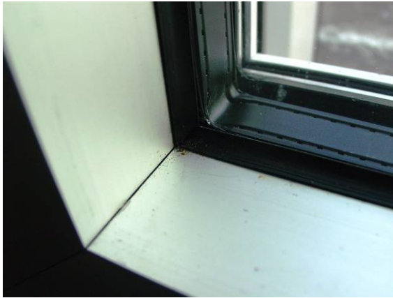
Fig. 5 Corner design of internal glazing gasket
